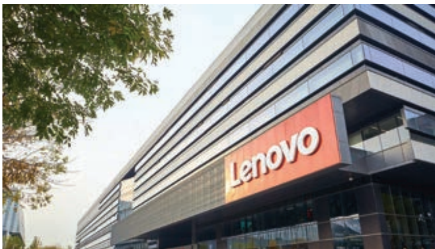
Lenovo's operation center in Beijing, China.
